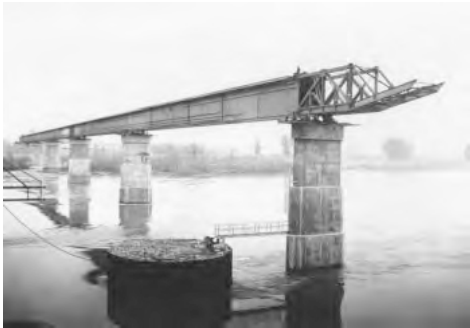
Figure 20.41c Leading end of north girder train is now supported on pier 5.
