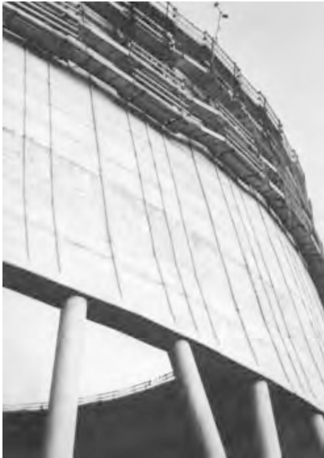
FIGURE 14.40: Column to lintel connection.
