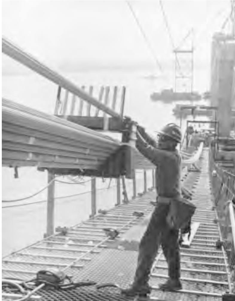
Figure 20.37b Cable formers maintain strand alignment in cables prior to compaction. Each finished cable is about 15-1/4 in. (387 mm) in diameter. (Courtesy of Bethlehem Steel Corporation.)
