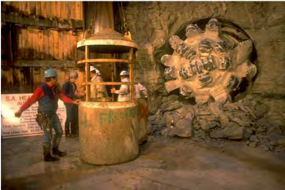
FIGURE 15B.13 Rock TBM holing through. (© David Sailors, 1988. With permission.)
