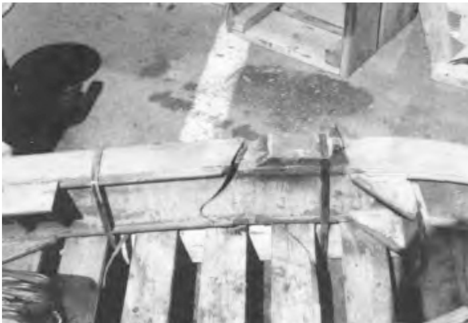
FIGURE 24.2: Fatigue cracking at welded detail in vehicle frame.
