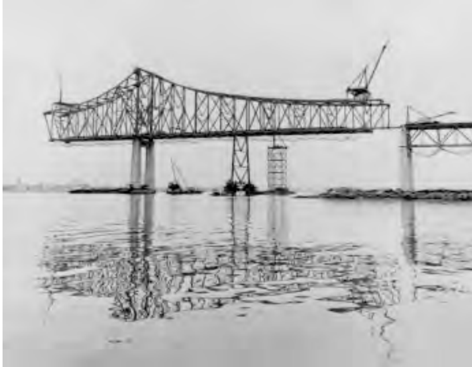
FIGURE 20.44: Closure of east side span, Commodore John Barry cantilever truss bridge, Chester, Pa., 1973. A high-tower derrick boat (in background) started erection of trusses at both main piers, supported on falsework; then erected top-chord travelers for main and side spans. The sidespan traveler carried steelwork erection to closure, as shown, and the falsework bent was then removed. The mainspan traveler then cantilevered the steelwork (without falsework) to midspan, concurrently with erection by the west-half mainspan traveler, and the trusses were closed at midspan. Commodore Barry has a 1644-ft (501-m) main span, the longest cantilever span in the U.S., and 822-ft (251-m) side spans. (Courtesy of Bethlehem Steel Corporation.)
