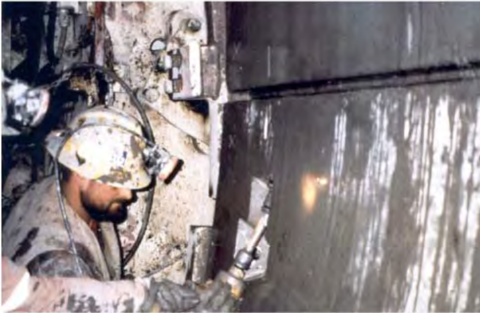
FIGURE 15B.15 Installation of one-pass liner. (© Bernie Martin. With permission.)
