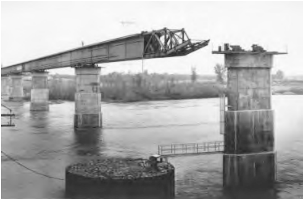
Figure 20.41a Leading end of north girder train moves across 250-ft (76-m) span 4, approaching pier 5. Main span is to right of pier 5.
