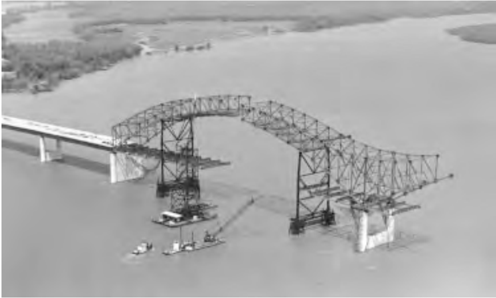
FIGURE 20.43: Erection of west arch span of twin-arch Hernando de Soto Bridge, Memphis, Tenn., 1972. The two 900-ft (274-m) continuous-truss tied-arch spans were erected by a high-tower derrick boat incorporating a pair of barges. West-arch steelwork (shown) was cantilevered to midspan over two pile-supported falsework bents. Projecting east-arch steelwork (at right) was then cantilevered to midspan (without falsework) and closed with falsework-supported other half-arch. (Courtesy of Bethlehem Steel Corporation.)
