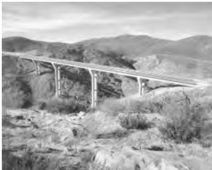
FIGURE 10.16b: Pine Valley Bridge, California. Construction completed. (From California Department of Transportation. With permission.)
