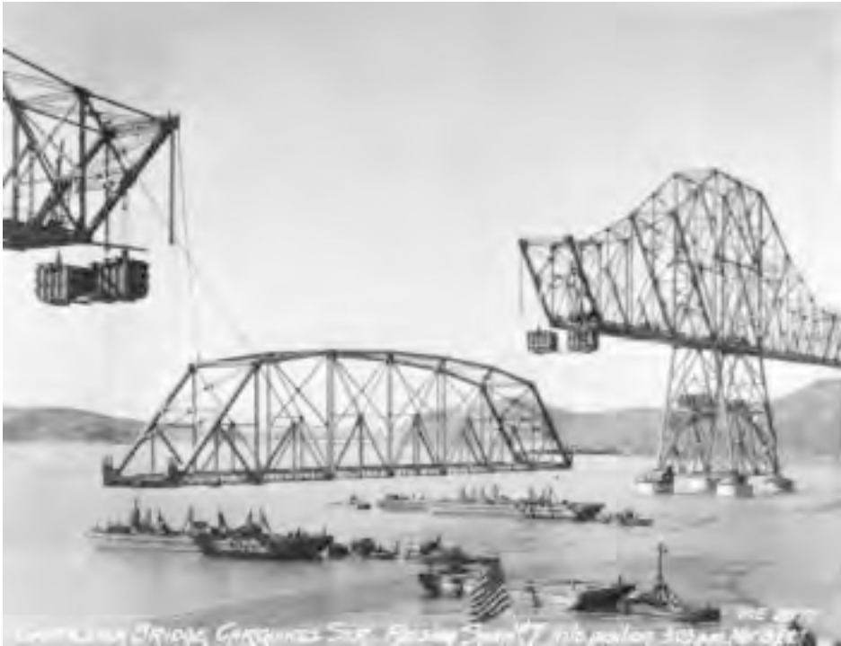
FIGURE 20.20: Raising of suspended span, Carquinez Strait Bridge, California, 1927. The 433-ft (132-m) suspended span, weighing 650 tons, was raised into position in 35 min., driven by four counterweight boxes having a total weight of 740 tons.
