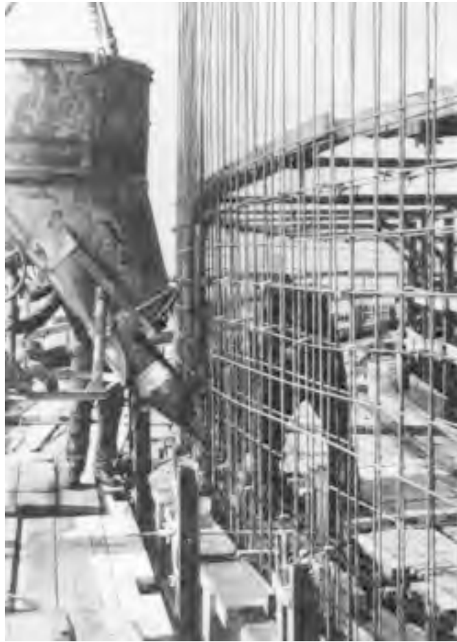
FIGURE 14.6 Steel reinforcement of shell wall.
