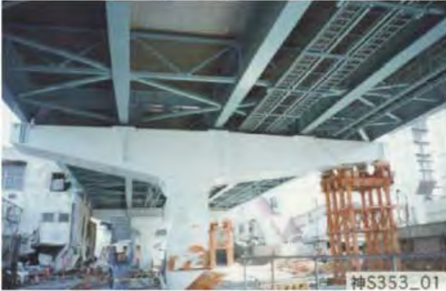
FIGURE 30.68 Collapsed building leaning against the Kobe Route 3 Expressway. (Courtesy of Hanshin Expressway Public Corporation.)
