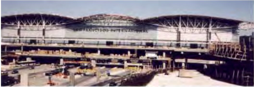
FIGURE 30.77 Construction of the new San Francisco Airport International Terminal. (Courtesy of Earthquake Protection Systems, Inc.)
