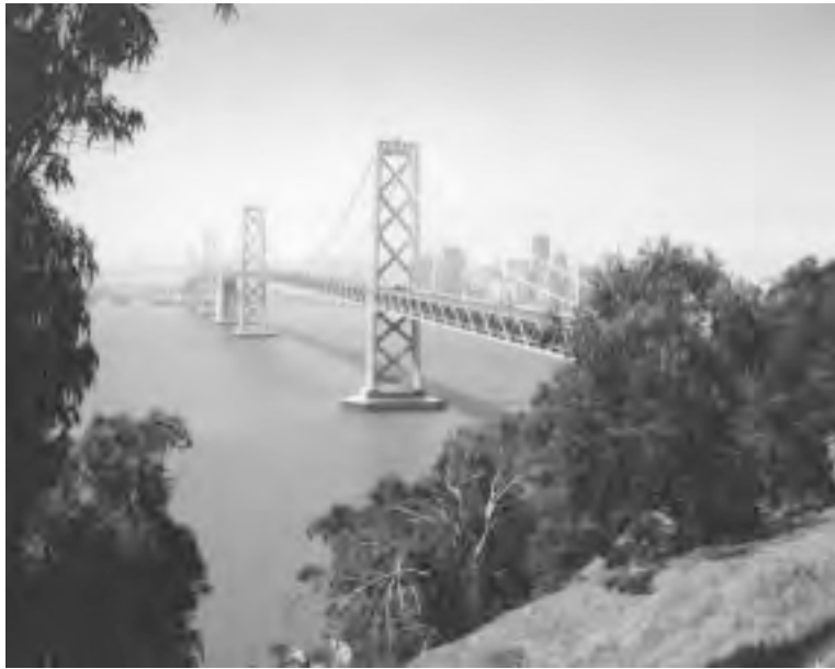
(a) West crossing spans.
