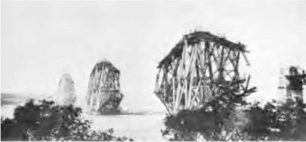
The massive cantilevers of the Forth bridge, shown under erection, were conceived in the shadow of the Tay bridge disaster.
