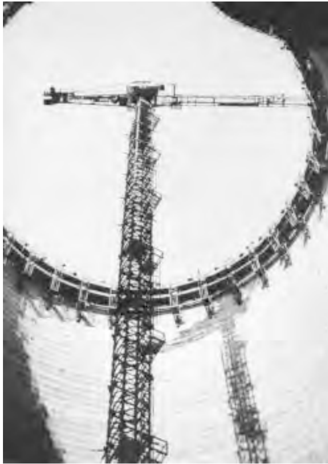
FIGURE 14.13: Attachments on shell wall.
