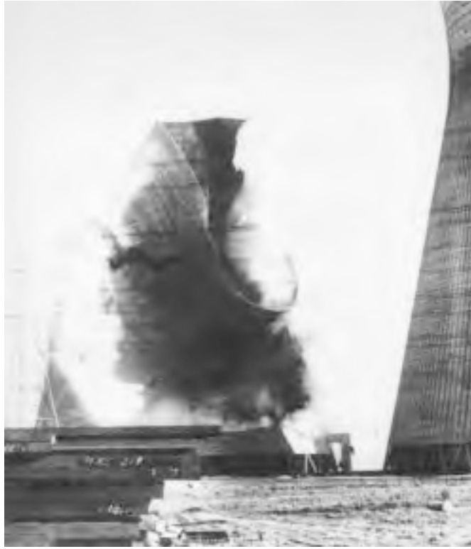
FIGURE 14.8: Collapse of Ferrisbridge Power Station shell.
