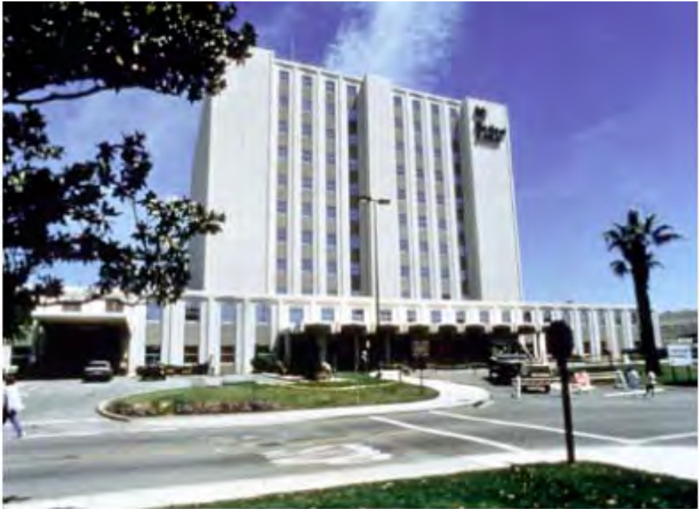
FIGURE 30.84 The existing Long Beach VA Hospital was seismically retrofitted with lead–rubber bearings. (Courtesy of Dynamic Isolation Systems, Inc.)
