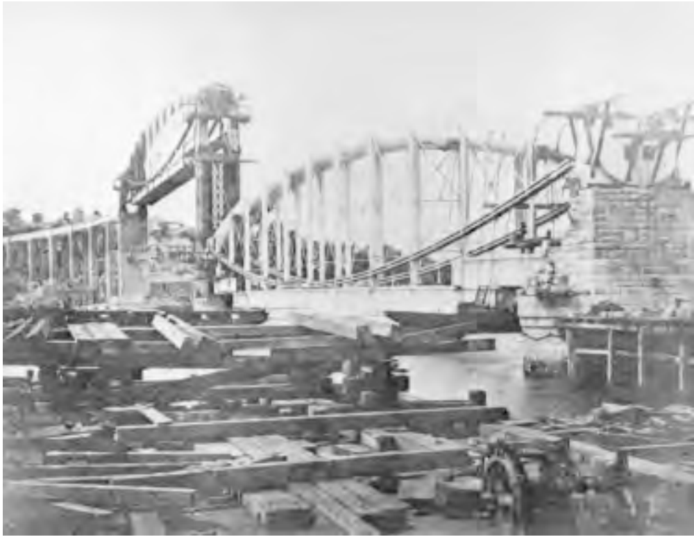
FIGURE 20.14: Royal Albert Bridge across River Tamar, Saltash, England, 1857. The two 455-ft (139-m) main spans, each weighing 1060 tons, were constructed on shore, floated out on pairs of barges, and hoisted about 100 ft (30 m) to their final position using hydraulic jacks. Pier masonry was built up after each 3-ft (1-m) lift.
