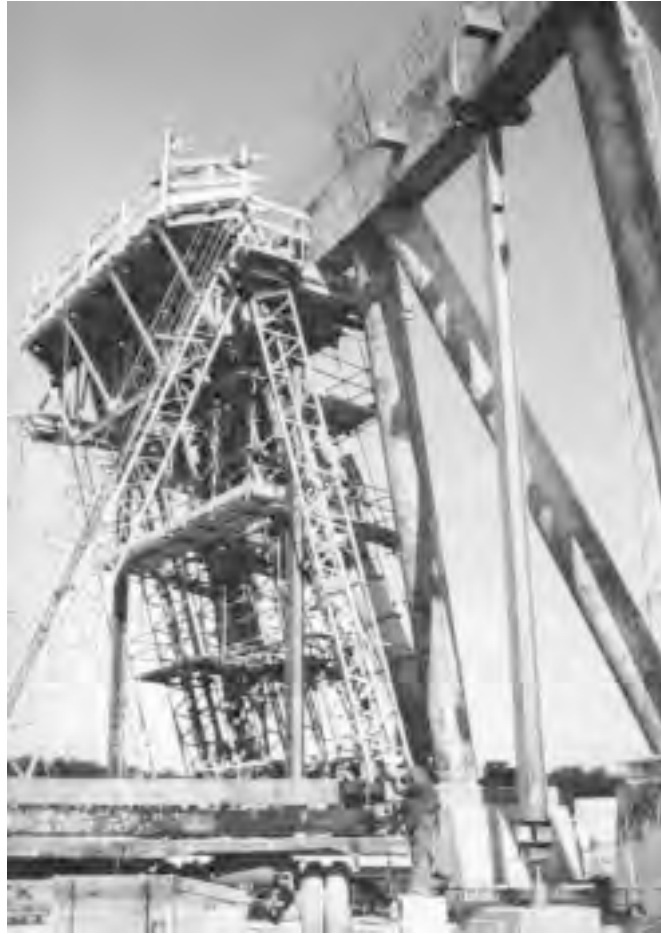
FIGURE 14.5: Fabrication of supporting columns.
