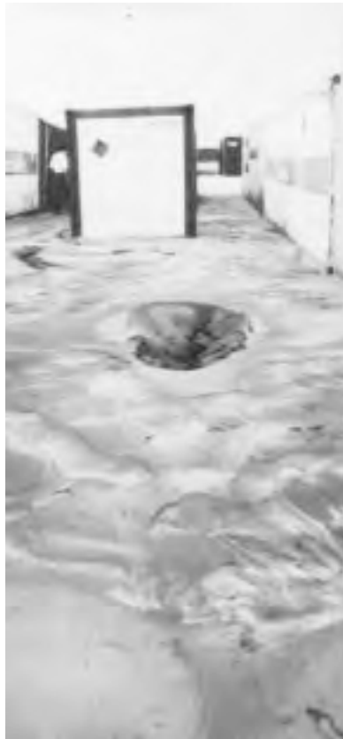
FIGURE 5.31: Photograph of sand boils.
