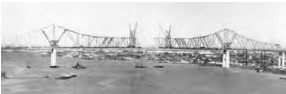
FIGURE 20.34: Greater New Orleans cantilever bridge, Louisiana, 1957. Tall double-boom deck travelers started at ends of main bridge and erected anchor spans on falsework, then the 1575-ft (480-m) main span by cantilevering to midspan. (Courtesy of Bethlehem Steel Corporation.)
