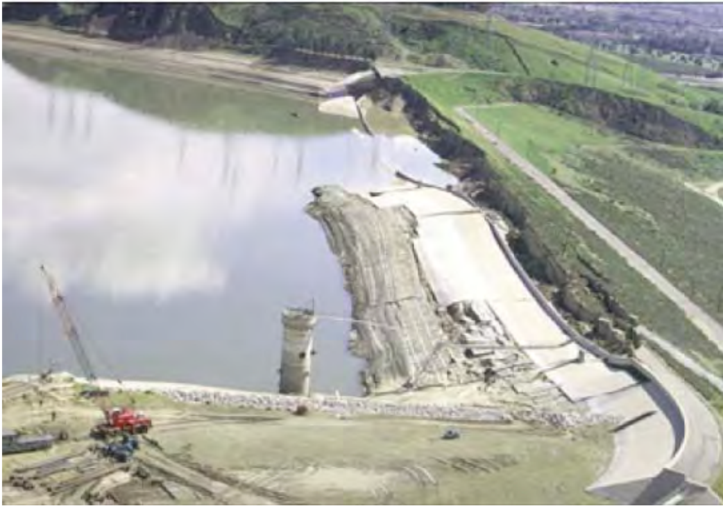
FIGURE 30.21 Damage to the Lower San Fernando Dam. (Courtesy of Steinbrugge Collection, Earthquake Engineering Research Center, University of California, Berkeley.)
