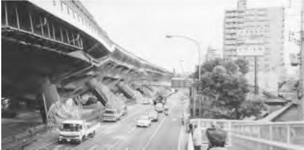
FIGURE 16.5: Collapsed Hanshin Expressway following the 1995 Kobe earthquake in Japan. (Photo by Mark Yashinsky. With permission.)
