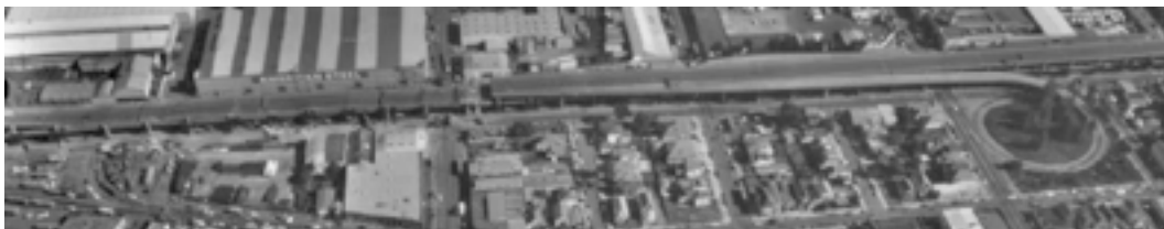
FIGURE 30.29 Aerial view of Cypress Street Viaduct showing collapse at north end (left) where the structure crossed over Bay mud, while the southern part (right), supported by dense sand, remained standing.
