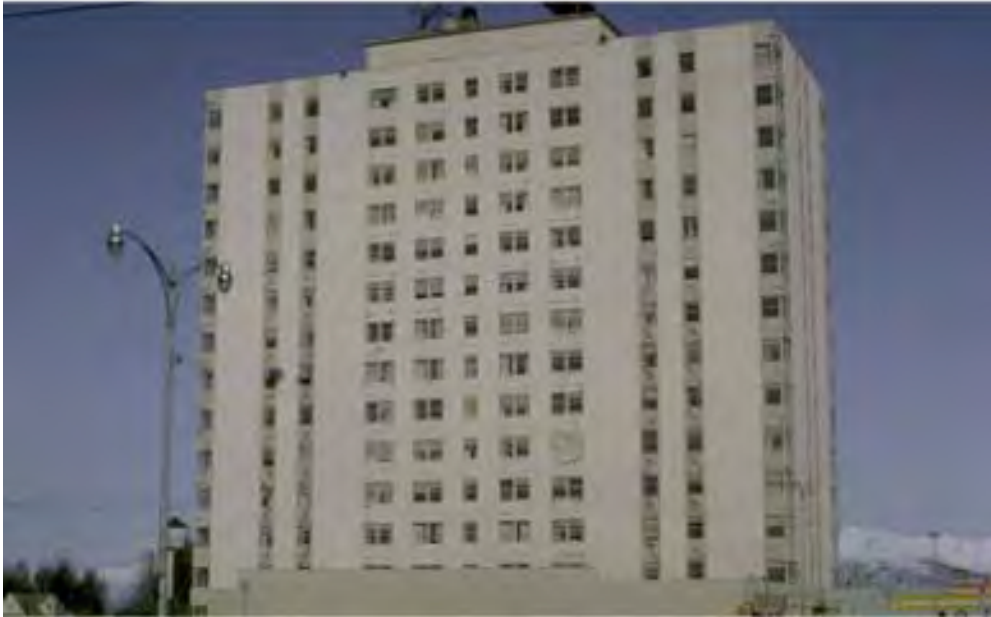
FIGURE 30.48 West elevation of Mt. McKinley Apartments after the 1964 Great Alaska earthquake. (Photograph by Karl Steinbrugge and courtesy of the Steinbrugge Collection, Earthquake Engineering Research Center, University of California, Berkeley.)
