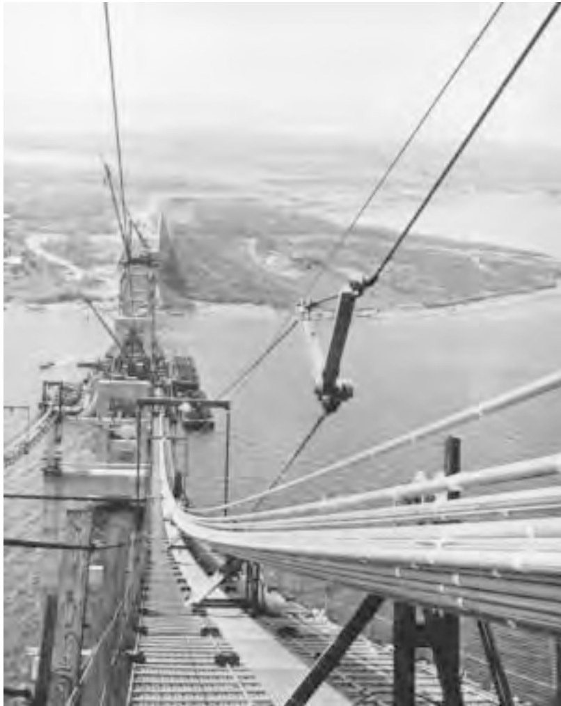
Figure 20.37a Aerial tramway tows PWS from west anchorage up side span, then on across other spans to east anchorage. Strands are about 1-3/4 in. (44 mm) in diameter.
