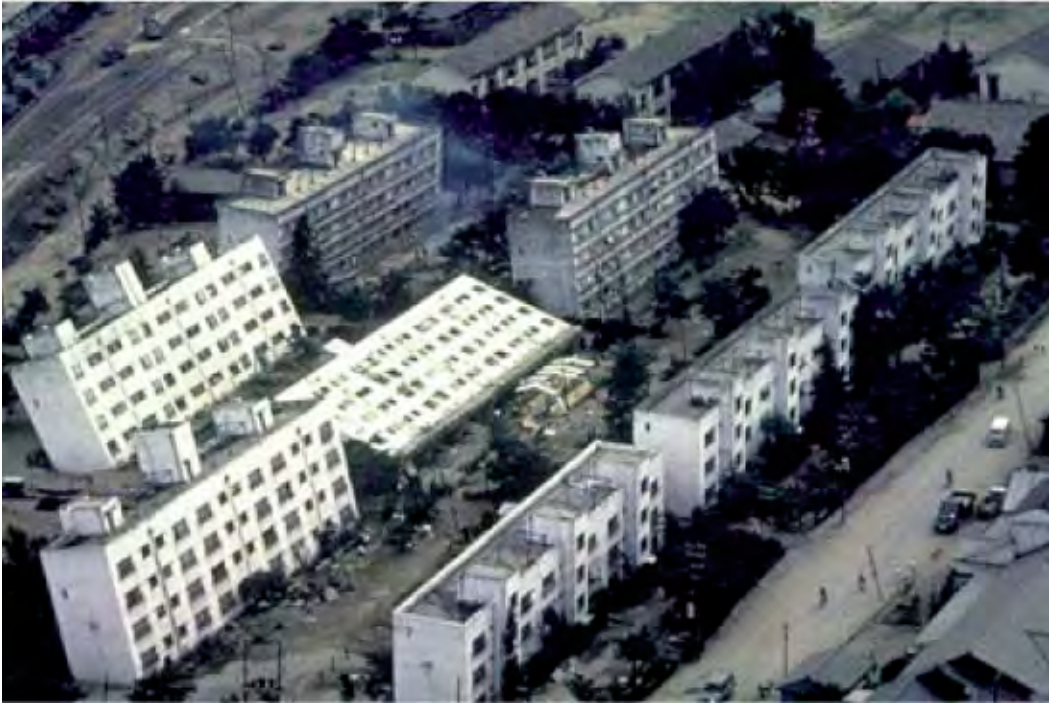
FIGURE 30.4 Liquefaction-caused building failure in Niigata, Japan. (Photograph by Joseph Penzien and courtesy of Steinbrugge Collection, Earthquake Engineering Research Center, University of California, Berkeley.)
