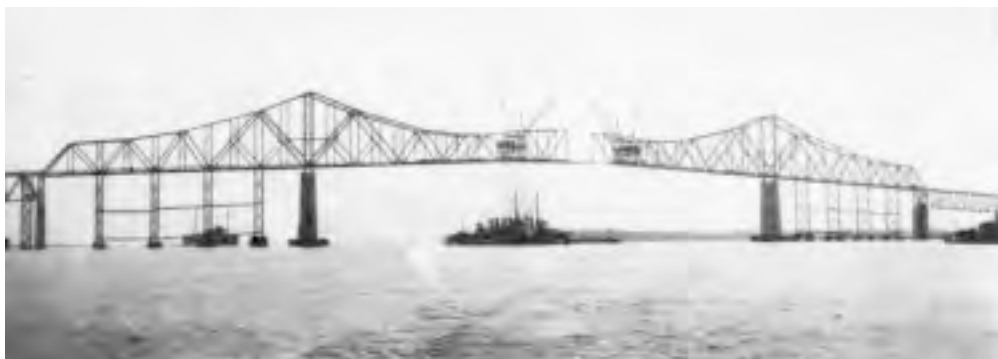
FIGURE 20.21: First Cooper River cantilever bridge, Charleston, S.C., 1929. Erection travelers constructed 450-ft (137-m) side spans on falsework, then went on to erect 1050-ft (320-m) main span (including 437.5-ft [133-m] suspended span) by cantilevering to midspan.
