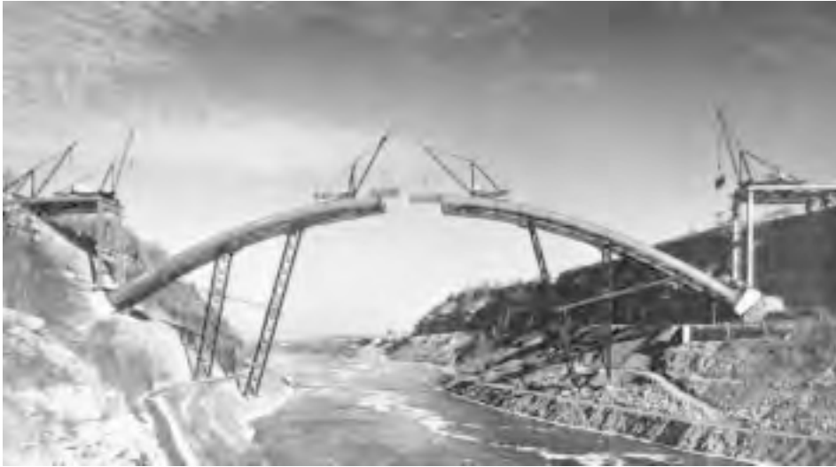
FIGURE 20.4: Lewiston-Queenston arch bridge, near Niagara Falls, New York, 1962. The world's longest fixed-arch span, at 1000 ft (305 m); rise is 159 ft (48 m). Box arch-rib sections are typically about 3 \times 13\text{-}1/2 ft ( 0.9 \times 4.1 m) in cross-section and about 44\text{-}1/2 ft (13.6 m) long. Job was estimated using erection tiebacks (same as shown in Figure 20.3), but subsequent studies showed the long, sloping falsework bents to be more economical (even if less secure looking). Much permanent steelwork was used in the falsework bents. Derricks on approaches load steelwork onto material cars that travel up arch ribs. The 115-ton-capacity travelers are shown erecting the last full-length arch-rib sections, leaving only the short, closing crown sections to be erected. Canada is at left, the U.S. at right. (Courtesy of Bethlehem Steel Corporation.)
