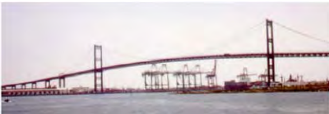
FIGURE 30.87 The Vincent Thomas Bridge, a three-span suspension structure built over the Port of Los Angeles.
