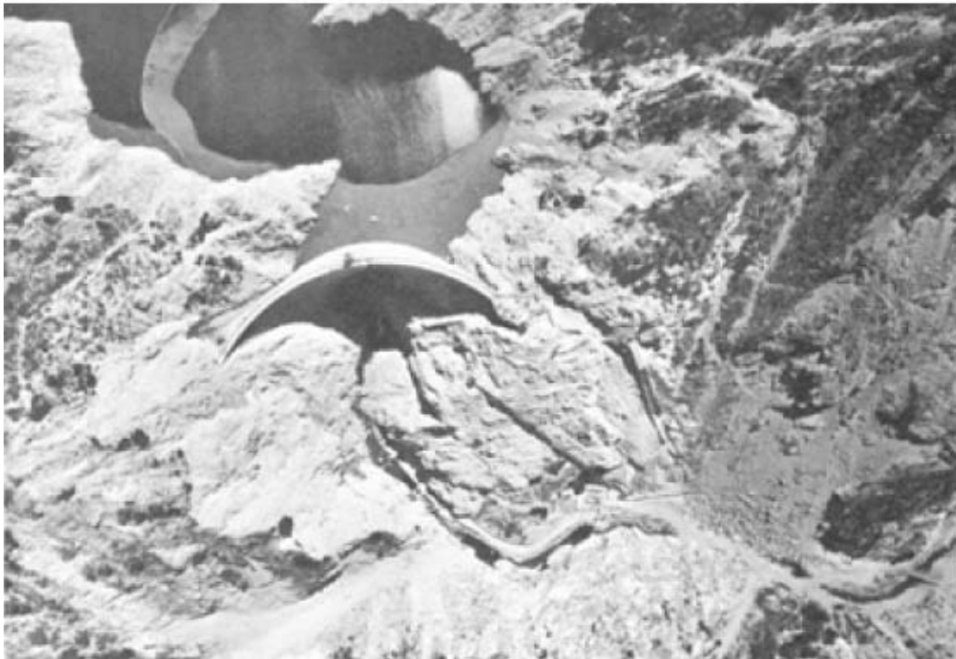
FIGURE 30.20 Landslides at Pacoima Dam following the 1971 San Fernando earthquake. (Courtesy of Steinbrugge Collection, Earthquake Engineering Research Center, University of California, Berkeley.)
