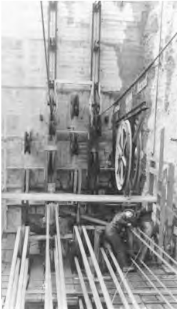
Figure 20.25b Tramway arrives at west anchorage. Wire loops shown in Figure 20.25a are removed from spinning wheels and placed around strand shoes at west anchorage. This tramway then returns empty to east anchorage, while tramway for other “leg” of endless hauling rope brings two wire loops across for second strand that is under construction for this cable.
