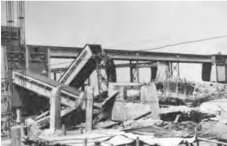
FIGURE 16.1: Collapsed elevated steel conveyor at Lujiatuo Mine following the 1976 Tangshan earthquake in China. (From California Institute of Technology, The Greater Tangshan Earthquake , California, 1996. With permission.)
