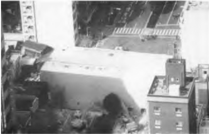
FIGURE 30.42 Eventual collapse of nine-story steel and reinforced-concrete (SRC) building after the Kobe earthquake. (Courtesy of NIST [9].)
