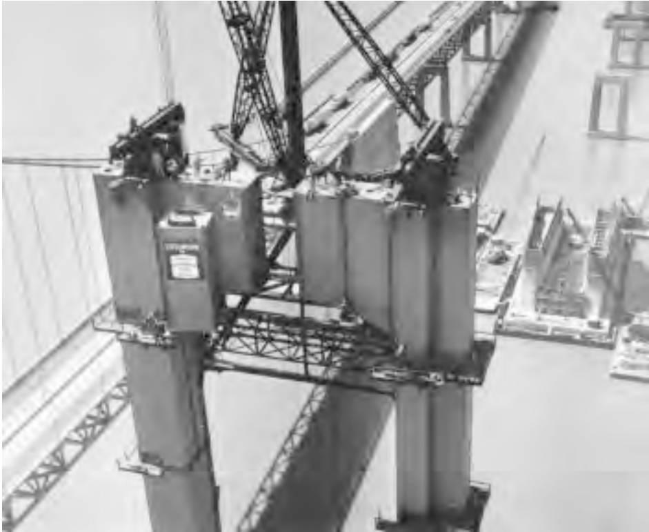
FIGURE 20.35: Tower erection, second Delaware Memorial Bridge, Wilmington, Del., 1966. The tower erection traveler has reached the topmost erecting position and swings into place the 23-ton closing top-strut section. The tower legs were jacked apart about 2 in. (50 mm) to provide entering clearance. The traveler jumping beams are in the topmost working position, above the cable saddles. The tower steelwork is about 418 ft (127 m) high. Cable anchorage pier is under construction at right. First Delaware Memorial Bridge (1951) is at left. The main span of both bridges is 2150 ft (655 m). (Courtesy of Bethlehem Steel Corporation.)
