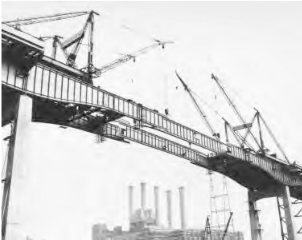
FIGURE 20.29: Erecting closing girder sections of Passaic River Bridge, New Jersey Turnpike, 1951. Huge double-boom travelers, each weighing 270 tons, erect closing plate girders of the 375-ft (114-m) main span. The closing girders are 14 ft (4.3 m) deep and 115 ft (35 m) long and weigh 146 tons each. Sidewise entry was required (as shown) because of long projecting splice material. Longitudinal motion was provided at one pier, where girders were jacked to effect closure. Closing girders were laterally stable without floor steel fill-in, such that derrick falls could be released immediately. (Courtesy of Bethlehem Steel Corporation.)
