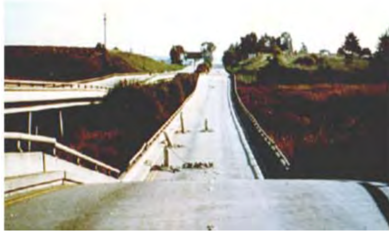
FIGURE 30.26 Piles penetrating the bridge deck.
