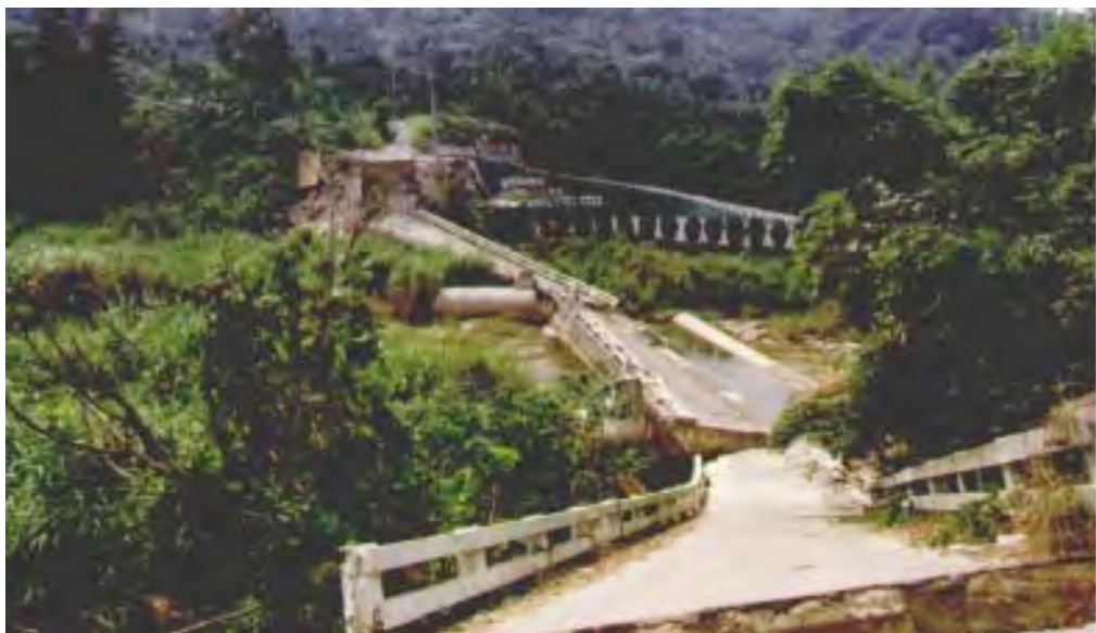
FIGURE 30.33 Three-span bridge rocked over during the 1999 Ji Ji, Taiwan earthquake.
