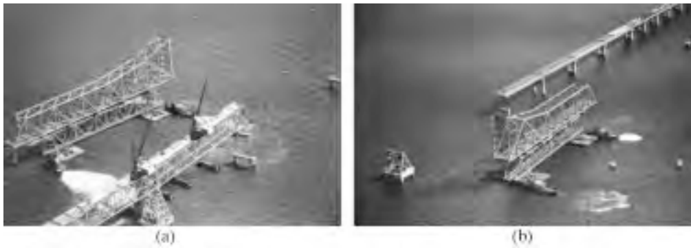
FIGURE 20.30: Floating-in erection of a truss span, first Chesapeake Bay Bridge, Maryland, 1951. Erected 300-ft (91-m) deck-truss spans form erection dock, providing a work platform for two derrick travelers. A permanent deck-truss span serves as a falsework truss supported on barges and is shown carrying the 470-ft (143-m) anchor arm of the through-cantilever truss. This span is floated to its permanent position, then landed onto its piers by ballasting the barges. (a) Float leaves erection dock, and (b) float arrives at permanent position. (Courtesy of Bethlehem Steel Corporation.)
