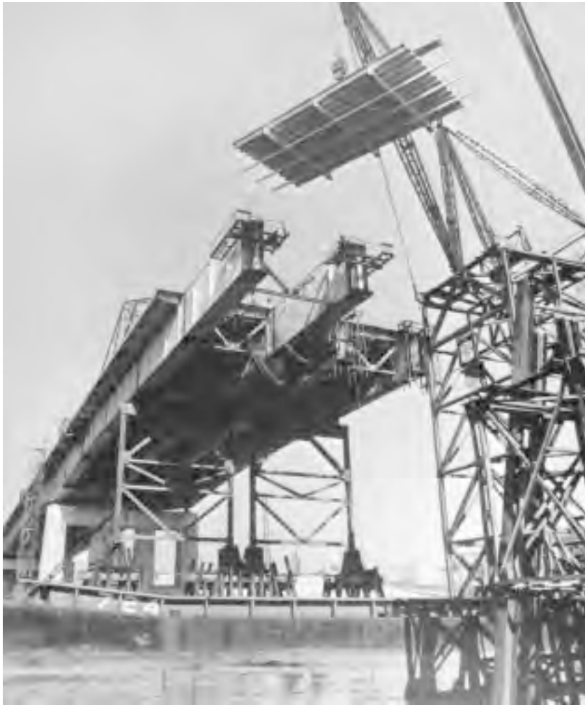
FIGURE 20.36: Erecting orthotropic-plate decking panel, Poplar Street Bridge, St. Louis, Mo., 1967. A five-span, 2165-ft (660-m) continuous box-girder bridge, main span 600 ft (183 m). Projecting box ribs are 5\text{-}1/2 \times 17 ft ( 1.7 \times 5.2 m) in cross-section, and decking section is 27 \times 50 ft ( 8.2 \times 15.2 m). Decking sections were field welded, while all other connections were field bolted. Box girders are cantilevered to falsework bents using overhead “positioning travelers” (triangular structure just visible above deck at left) for intermediate support. (Courtesy of Bethlehem Steel Corporation.)
