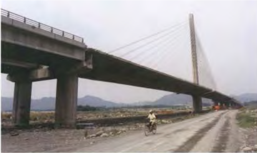
FIGURE 30.44 The Ji Lu cable-stayed bridge after the 1999 Taiwan earthquake.
