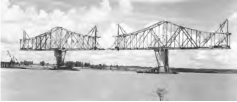
FIGURE 20.23: Balanced-cantilever erection, Governor O.K. Allen railway/highway cantilever bridge, Baton Rouge, La., 1939. First use of long balanced-cantilever erection in the U.S. On each pier 650 ft (198 m) of steelwork, about 4000 tons, was balanced on the 40-ft (12-m) base formed by a sloping falsework bent. The compression load at the top of the falsework bent was measured at frequent intervals and adjusted by positioning a counterweight car running at bottom-chord level. The main spans are 848-650-848 ft (258-198-258 m); 650 ft span shown. (Courtesy of Bethlehem Steel Corporation.)
