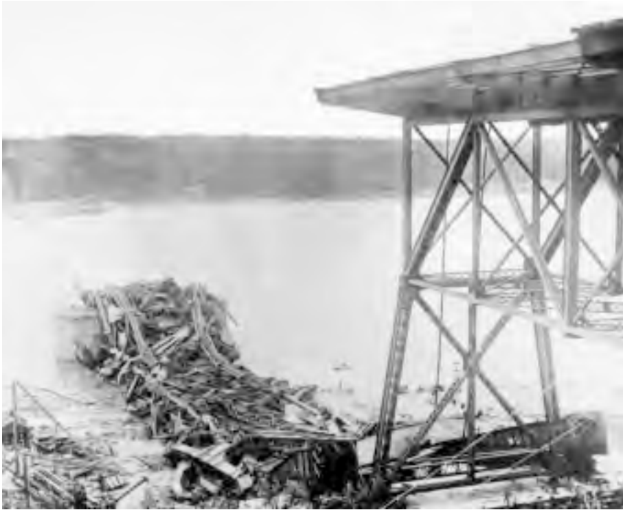
FIGURE 20.12: Wreckage of south anchor span of first Quebec railway cantilever bridge, 1907. View looking north from south shore a few days after collapse of 29 August 1907, the worst disaster in the history of bridge construction. About 20,000 tons of steelwork fell into the St. Lawrence River, and 75 workmen lost their lives.
