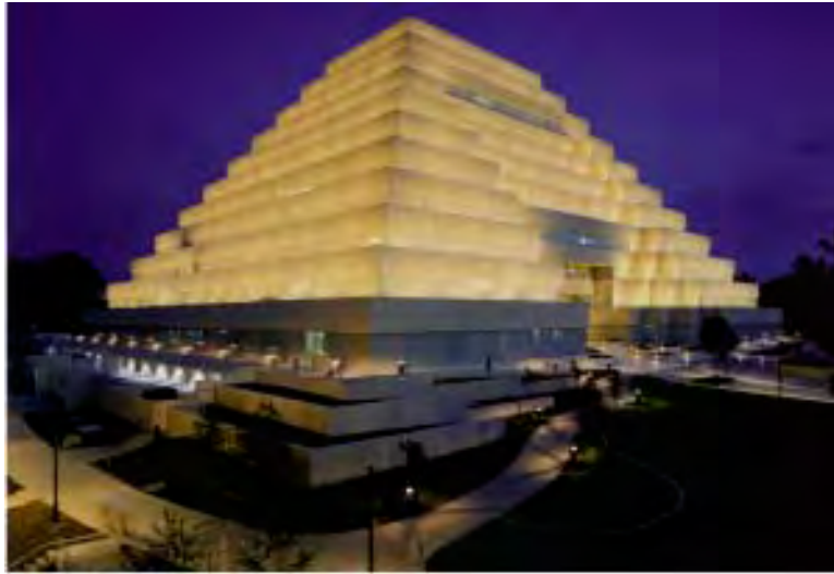
FIGURE 30.81 The uniquely shaped Money Store was designed with fluid viscous dampers to improve its seismic behavior. (Courtesy of Marr-Shaffer & Miyamoto, Structural Engineers.)
