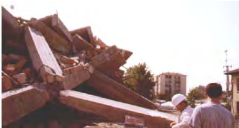
FIGURE 30.59 Collapsed reinforced-concrete building during the 1999 Kocaeli earthquake.
