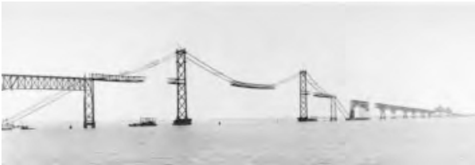
FIGURE 20.6: Suspension spans of first Chesapeake Bay Bridge, Maryland, 1952. Deck steelwork is under erection and is about 50% complete. A typical four-panel through-truss deck section, weighing about 100 tons, is being picked in west side span, and also in east side span in distance. Main span is 1600 ft (488 m) and side spans are 661 ft (201 m); towers are 324 ft (99 m) high. Cables are 14 in. (356 mm) in diameter and are made up of 61 helical bridge strands each (see Figure 20.8).
