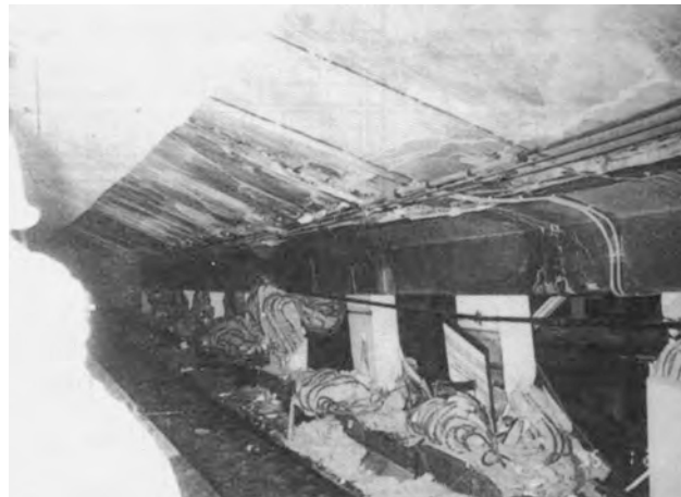
FIGURE 30.53 Flexural damage to columns at lower-level of Dakkai Subway during the 1995 Kobe earthquake. (Courtesy of Japan Society of Civil Engineers [5].)
